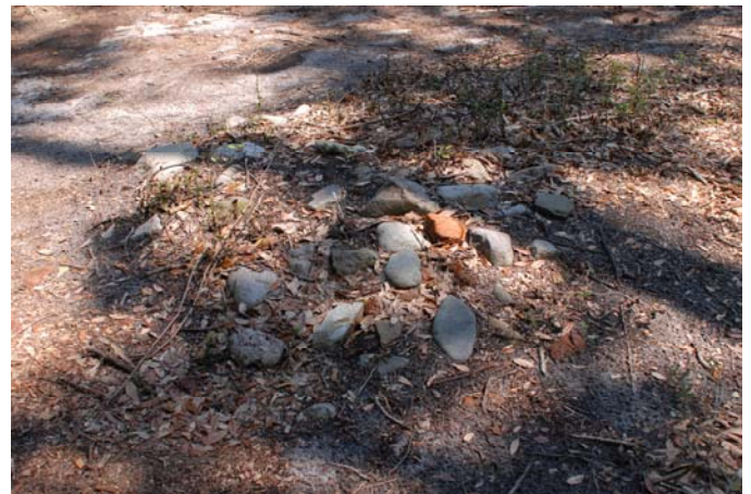
Figure 2. Piles of handmade brick and ballast stones of varied sizes, likely taken from colonial household ruins during the construction of Fort Anderson, were above-ground signatures of Civil War era barracks chimney falls. Photo by the author.
