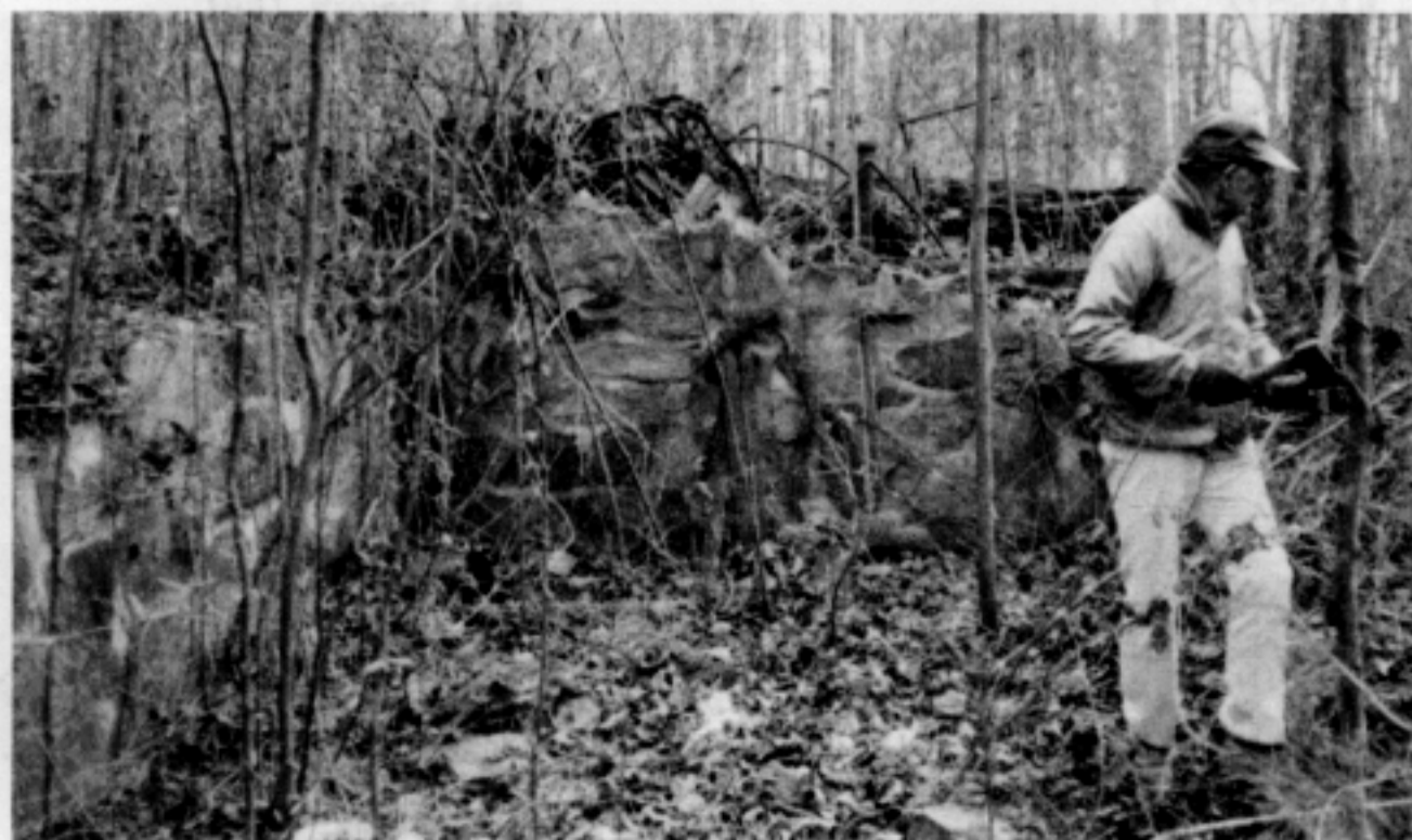
Stone walls of basement addition to McGregor summer house
