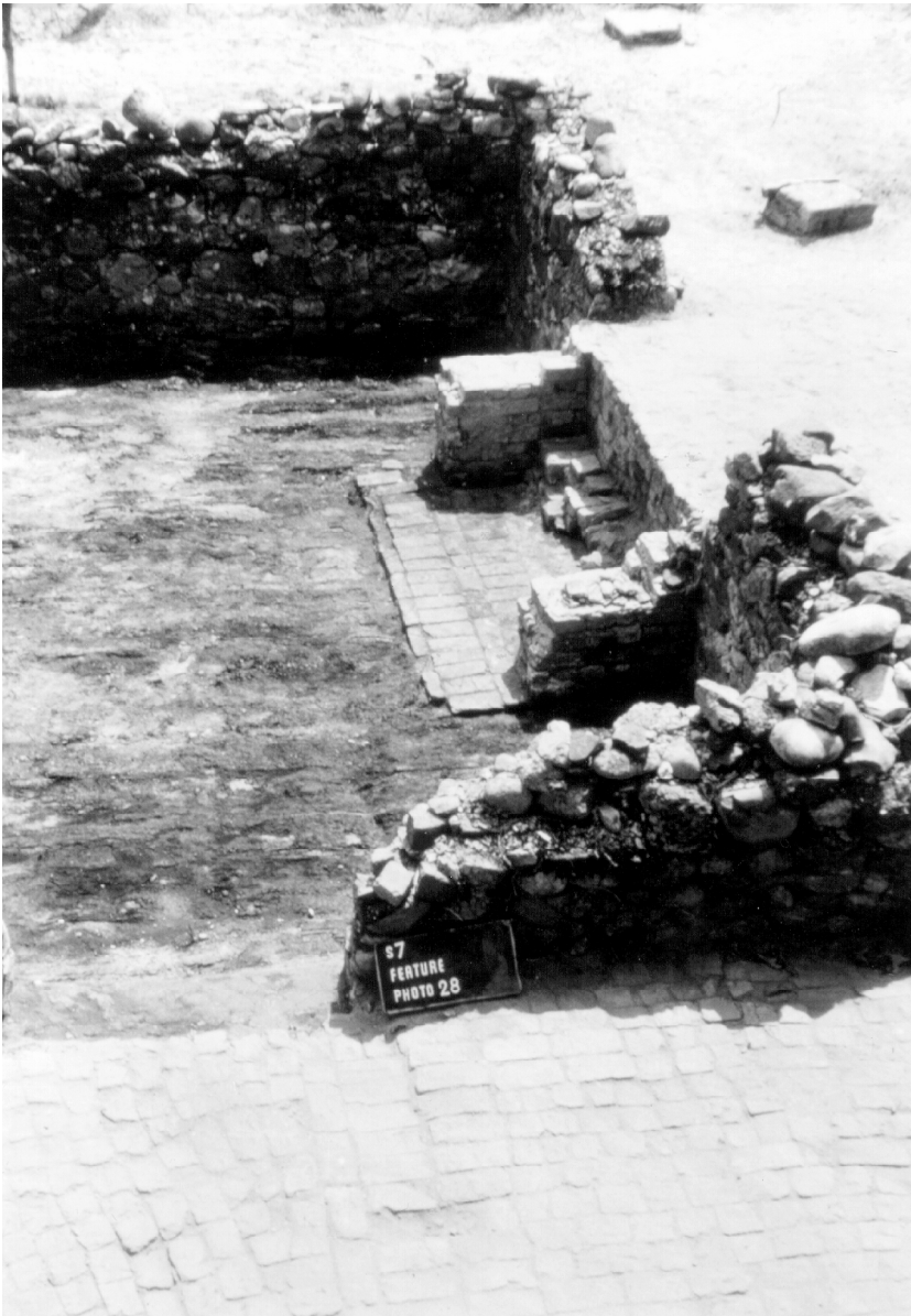
Figure 7. Archaeological investigations of the domestic ruins at Brunswick Town revealed many architectural details of the former residences. For example, this photograph of the excavated Hepburn-Reonalds ruin illustrates a ballast stone foundation, with hand-made bricks used for the chimney, a terrace, and pier supports for a porch. The remains of burned planking from a wooden floor are also visible. Courtesy of Historic Sites Section, North Carolina Department of Cultural Resources.
