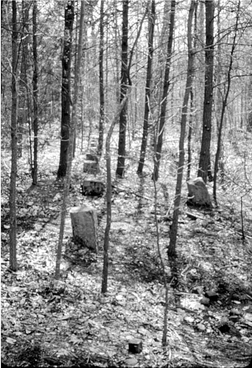
Figure 3. South-facing view of granite piers of the Mountain View Hotel/Linwood College dormitory. These are the eastern piers supporting the rear of the building. Note the chimney fall in the middle right.
