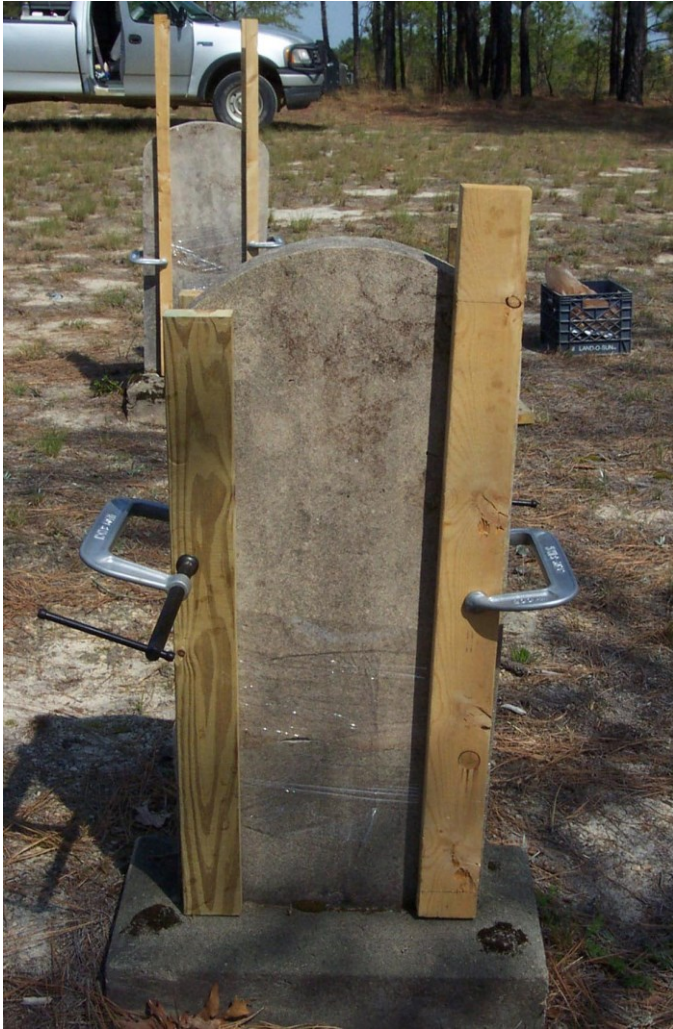
Figure 6. Example of major stone repairs using epoxy bonding and supportive clamps.
