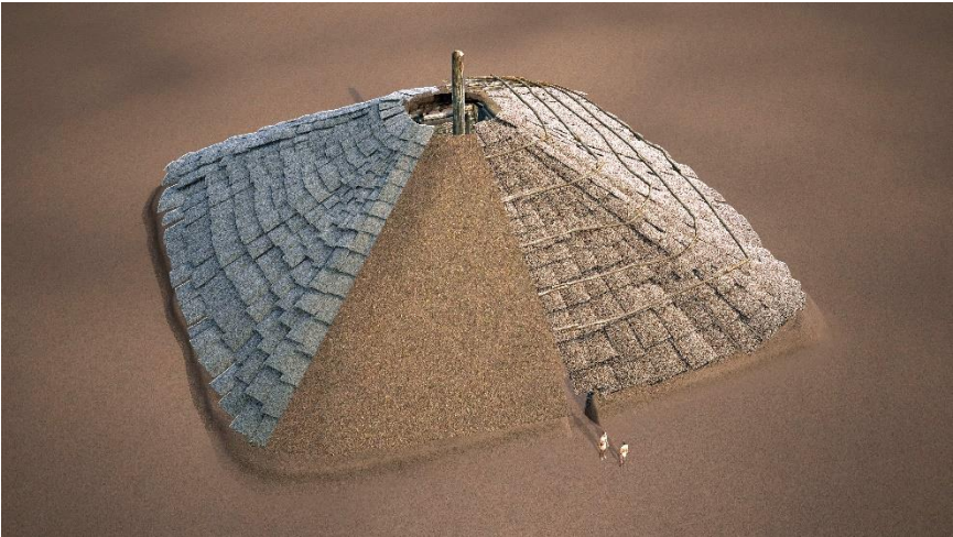
Figure 12. Cutaway of model showing bark, earth, and bark coverings.
