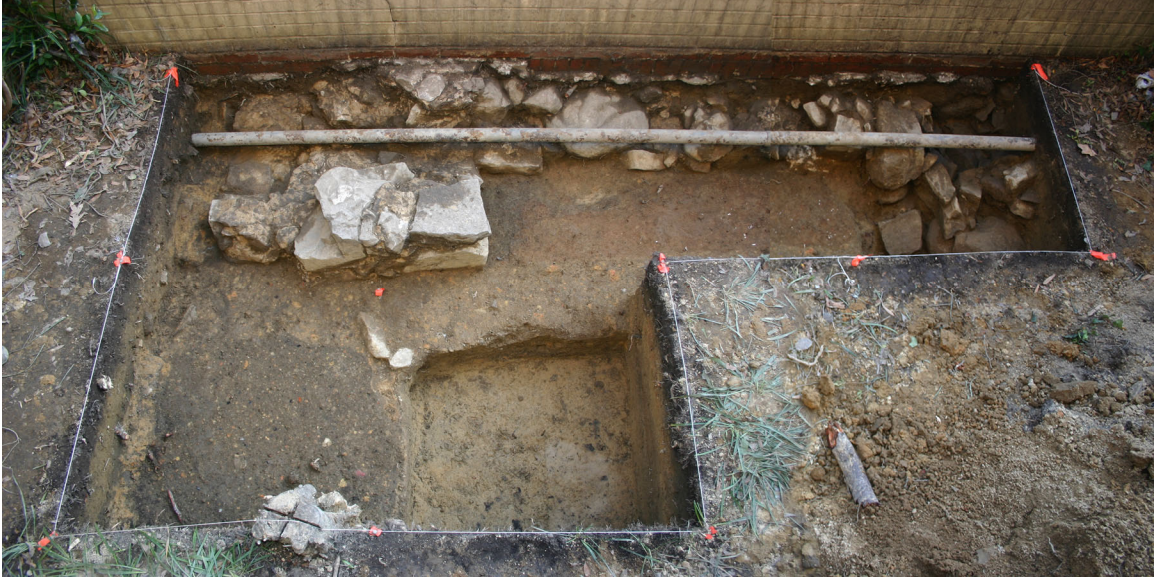
Figure 21. Composite photograph of the completed excavation, showing the southeast corner column foundation (at left) and the adjacent interior column foundation (at right). View to the south.
