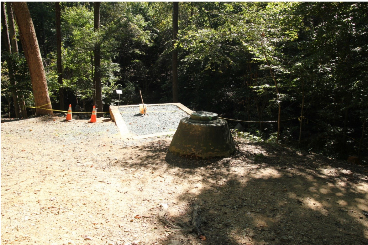
Figure 10. South facing view of the brick-and-concrete manhole and upper concrete tank, both elements of Component 5, at the northern edge of the site.
