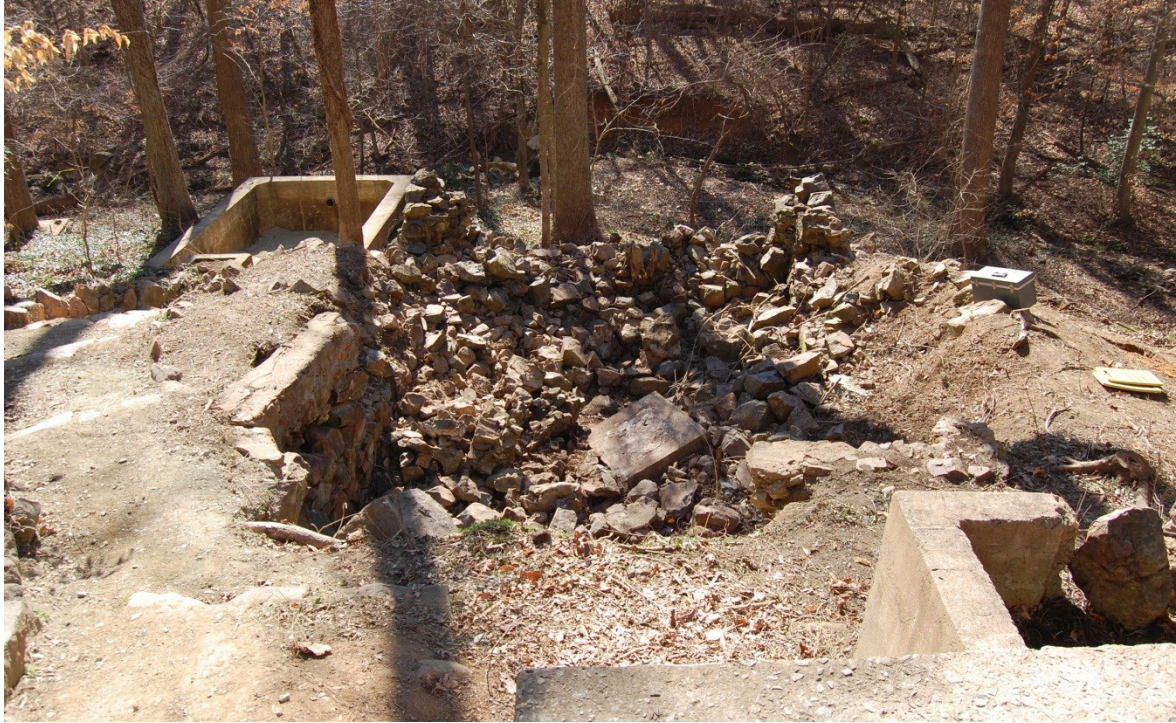
Figure 6. View of Component 3, taken from northern (upper) concrete tank facing south. Photographed in February 2012, prior to removal of the collapsed stone debris overlying the structure's floor. The southern (lower) concrete tank, part of Component 5, is visible in the top left of background.
