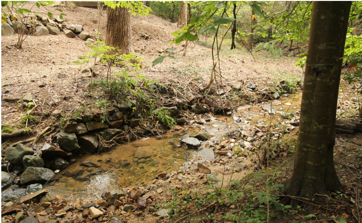
Figure 5. View of Component 2. Partially intact stacked stone retaining wall present in the bank of Battle Branch Creek directly south of sludge bed. Photograph taken from southern bank of creek, facing approximately east.
