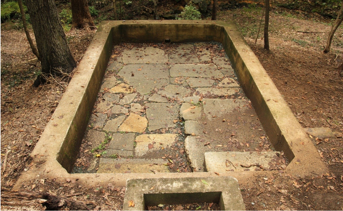
Figure 11. South facing view of southern (lower) concrete tank (Component 5). The small concrete junction box, also part of Component 5, is partially visible at the bottom of the image.
