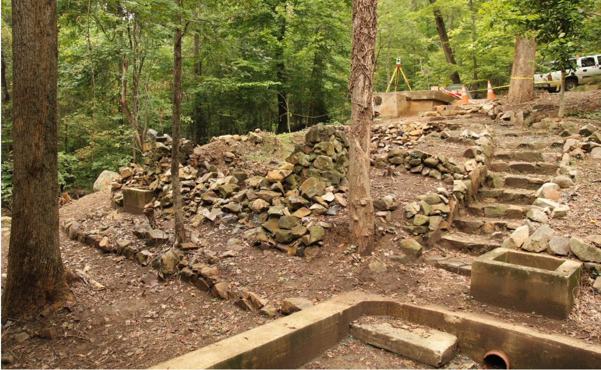
Figure 9. General view of site, facing northwest from the lower concrete tank (foreground). Other Component 5 elements include the small concrete junction boxes (at bottom right and left, adjacent to Component 4 rubble), and the northern (upper) concrete tank with the total station resting atop it.
