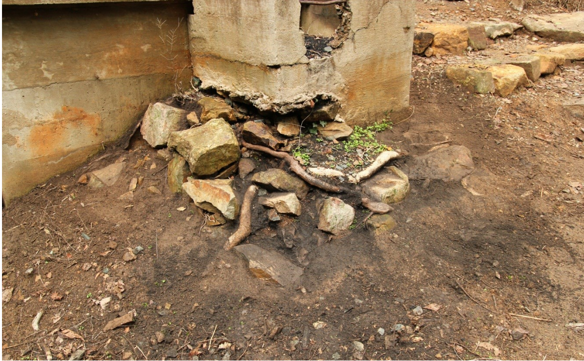
Figure 8. View of the western end of Component 4, lying beneath the small concrete junction box poured against the southern edge of the upper concrete tank (Component 5). View to northeast.
