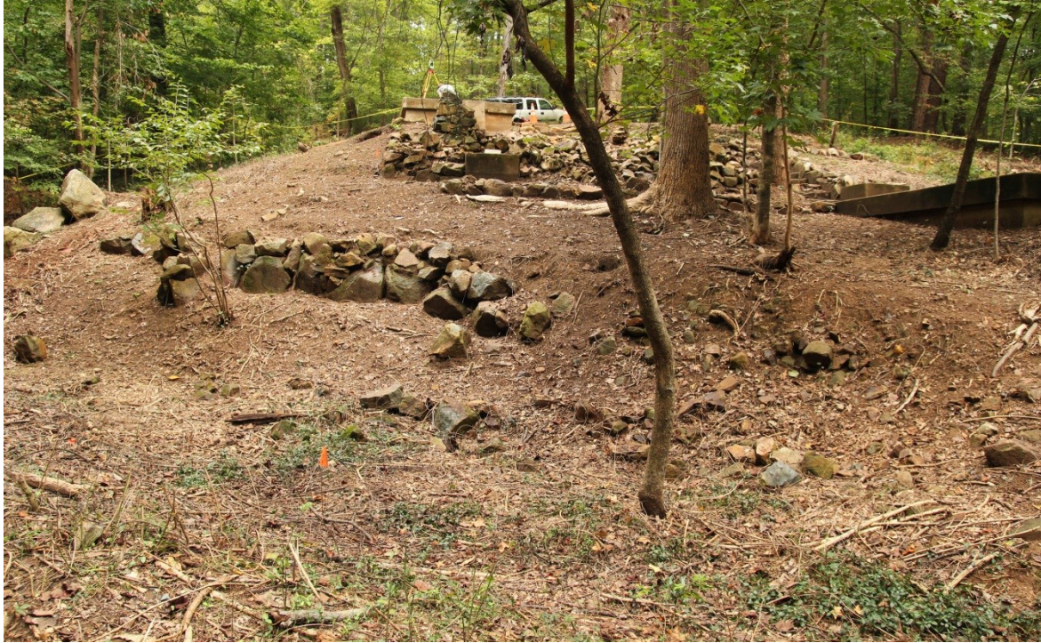
Figure 4. View of Component 2. The stacked stone retaining wall and northern edge of the sludge bed runs midway across the image. Halfway across from the left, the wall is collapsed into the sludge bed basin. Photograph taken from bank of Battle Branch Creek, facing north.
