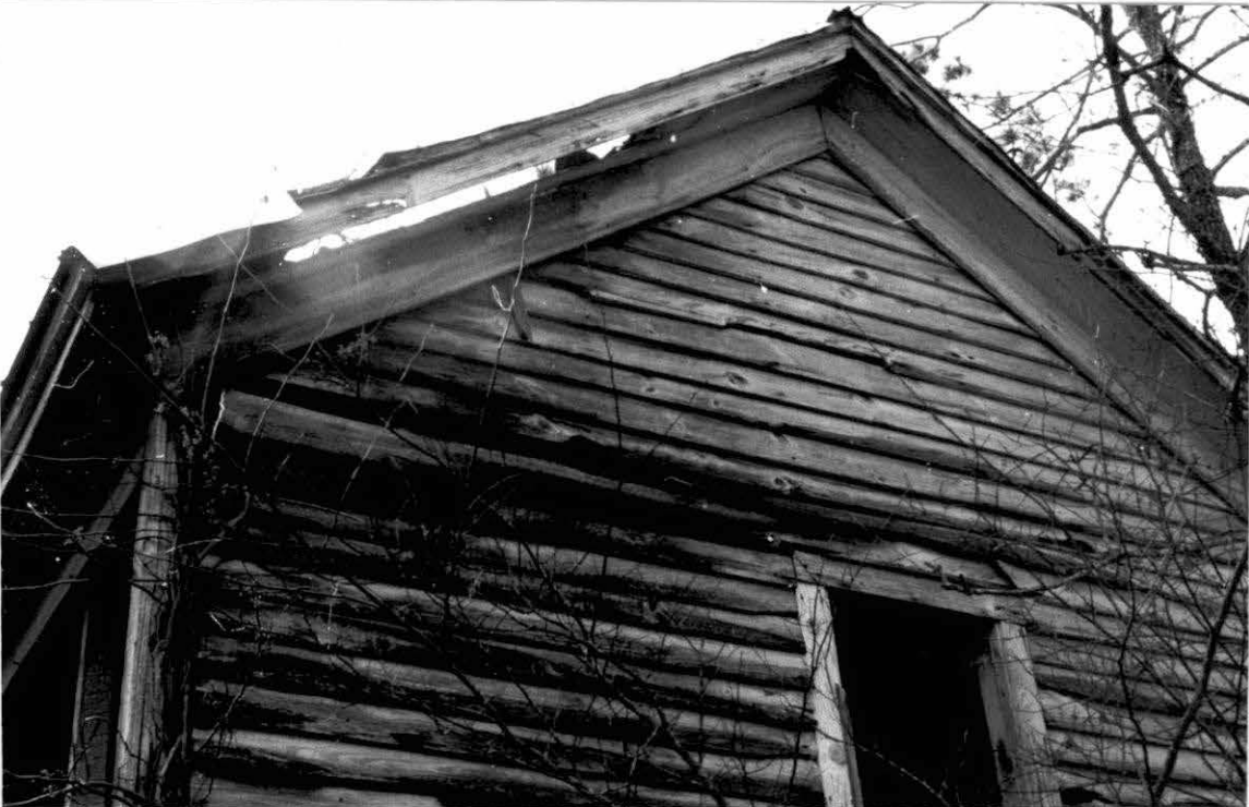
Figure 10. Close-up View of Frame House at 31Wa673, Showing Detail of Siding and Boxed Soffit.
